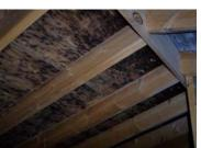
Indoor Air Quality Testing indicated elevated levels of mold and in the home the tape lifts verified hypoallergenic mold in the attic growing on the sheathing.
