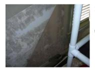
Indoor Air Quality Testing indicated elevated levels of mold and further investigation uncovered potentially toxigenic mold mold behind wall paper.
